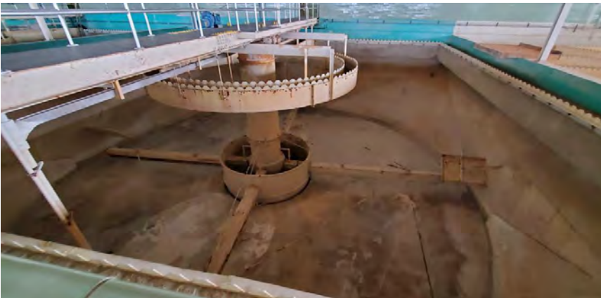
Photo 5: Solids Contact Basin 2
