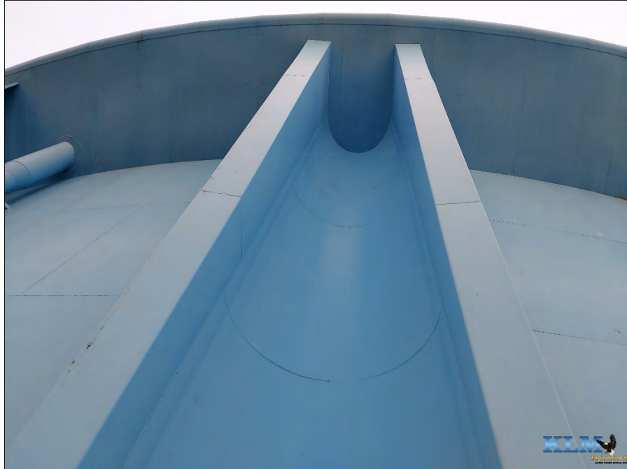
Photo No. 27 Shell exterior conditions
