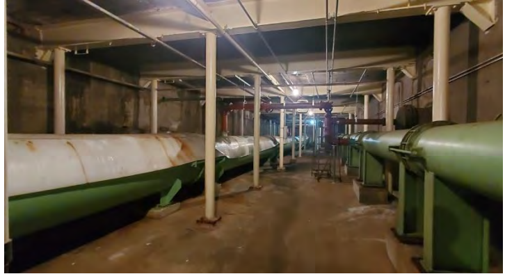
Photo 22: Transmission Main Tunnel
