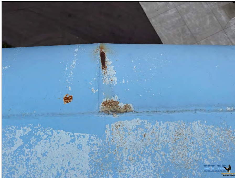
Photo No. 22 Coating conditions on roof
