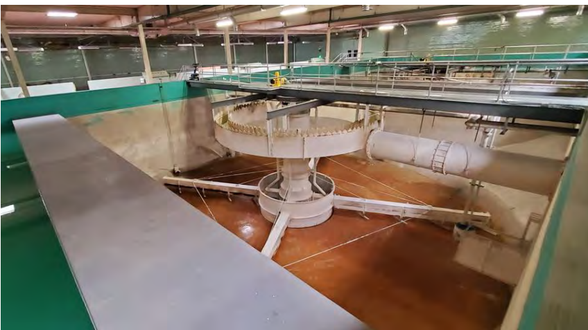
Photo 6: Solids Contact Basin 5
