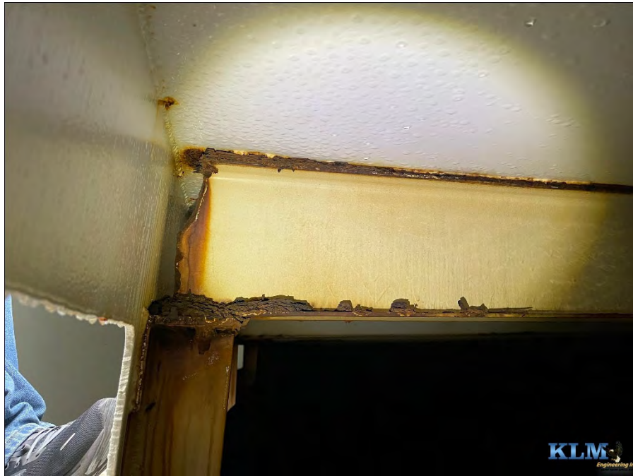
Photo No. 9 Typical roof rafter to shell connection
