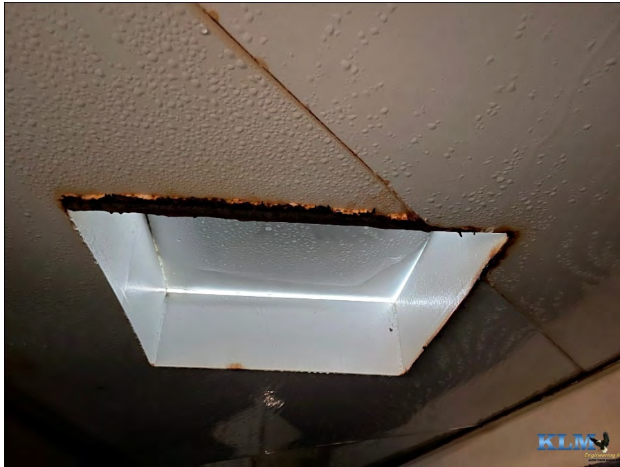
Photo No. 4 Manway access on roof
