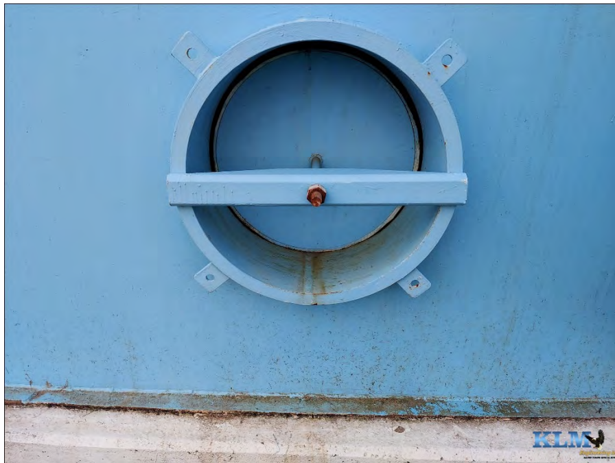
Photo No. 32 Manway on shell exterior
