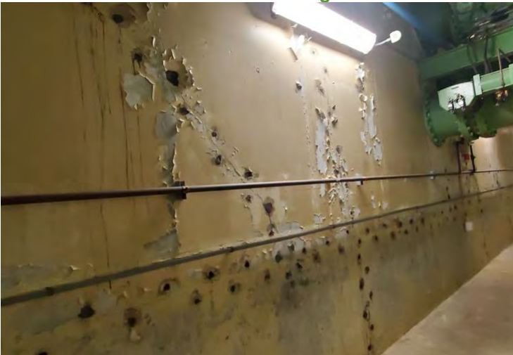
Photo 12: Filter Gallery (Filters 1 - 10) – Concrete Wall Repairs
