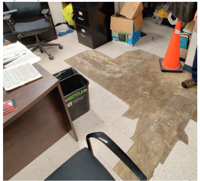
Photo 24: Operations Supervisor Office - Flooring
