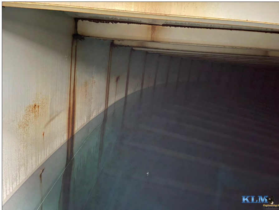
Photo No. 14 Shell conditions
