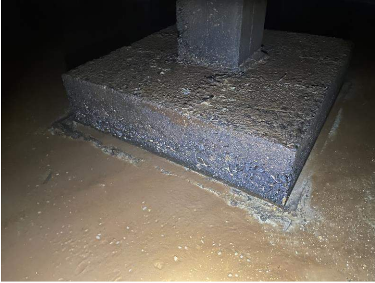
Figure 10 Spalling at concrete column pedestal
