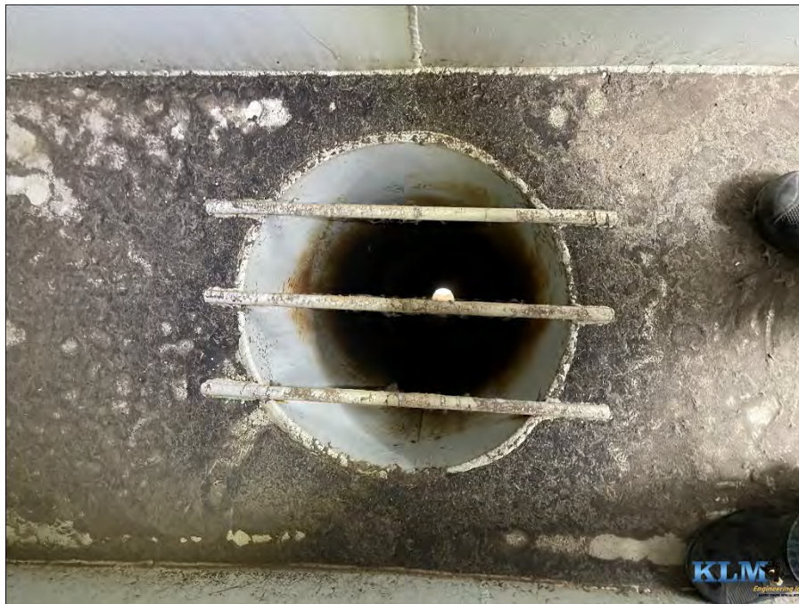
Photo No. 12 Overflow pipe condition
