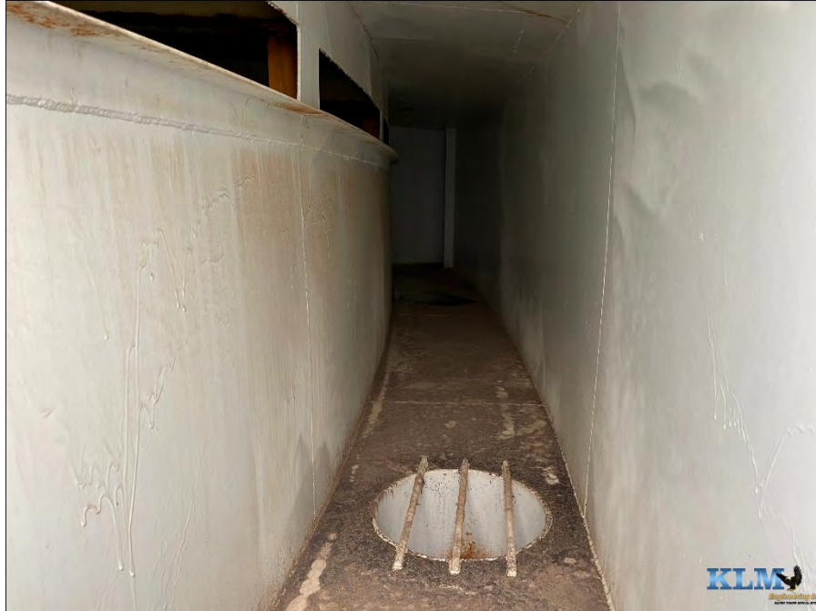
Photo No. 11 Overflow corridor
