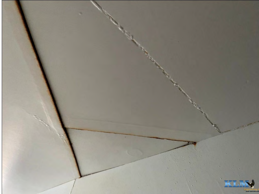
Photo No. 5 Condition of roof plates
