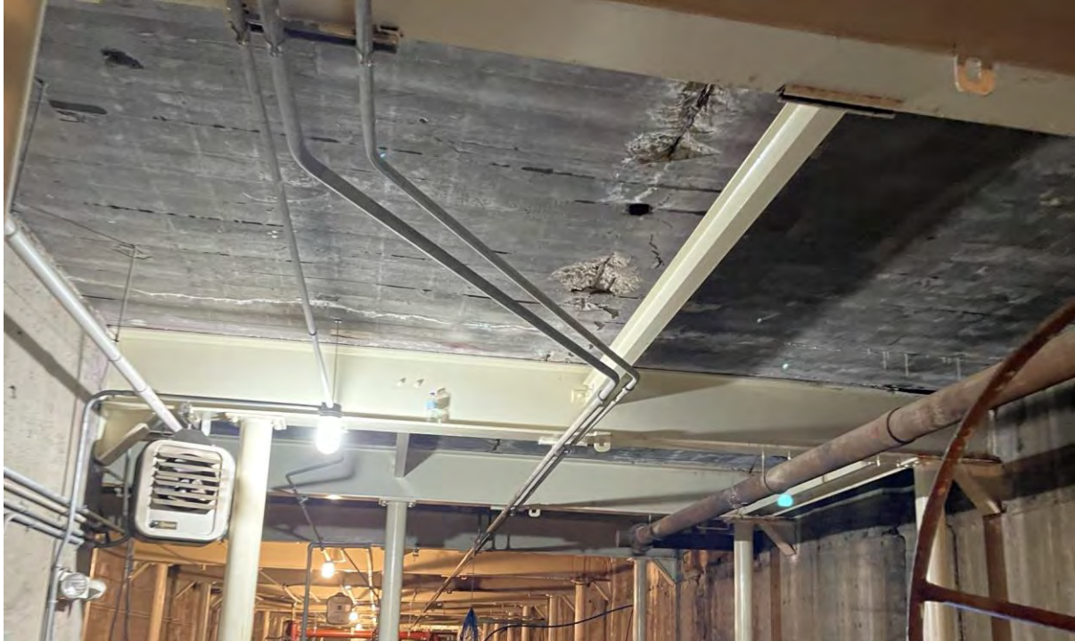
Figure 1. Existing Concrete Decking
