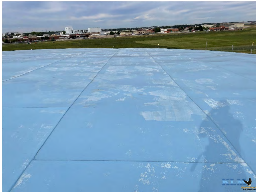
Photo No. 21 Roof conditions
