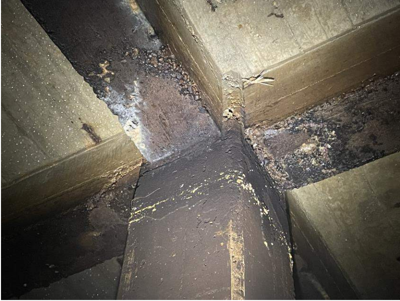
Figure 8 Unconsolidated concrete and exposed aggregate
