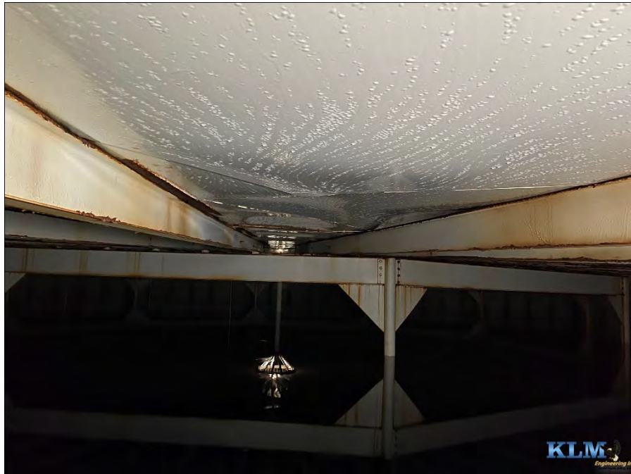
Photo No. 6 Condition of roof and rafters
