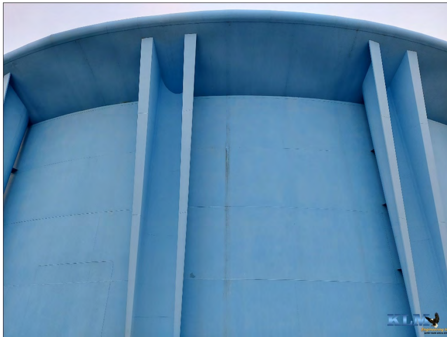
Photo No. 28 Shell exterior conditions
