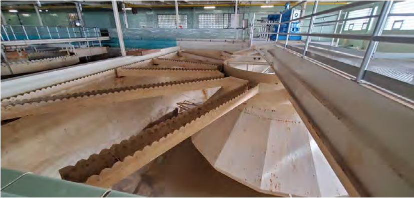
Photo 4: Solids Contact Basin 1
