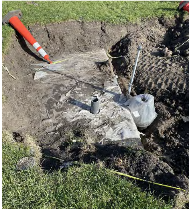
Figure 2 Exposed exterior of roof slab
