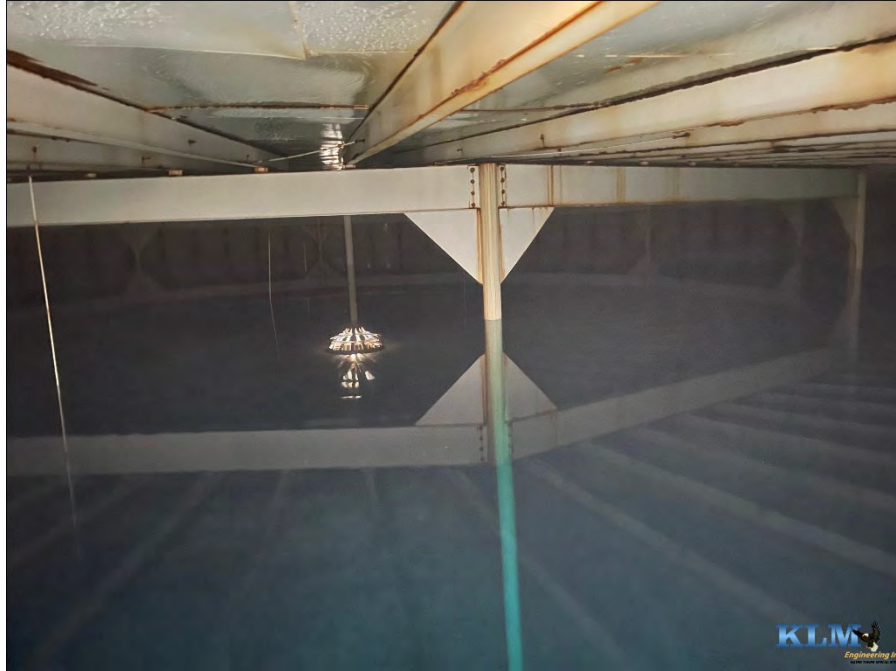
Photo No. 3 Interior conditions
