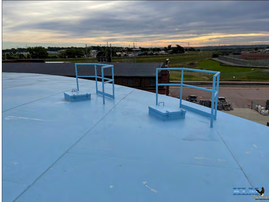
Photo No. 17 Roof and manways conditions
