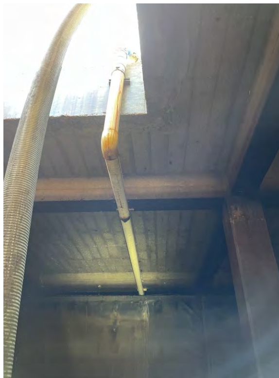
Figure 23 Drain pipe (end/exterior connection)
