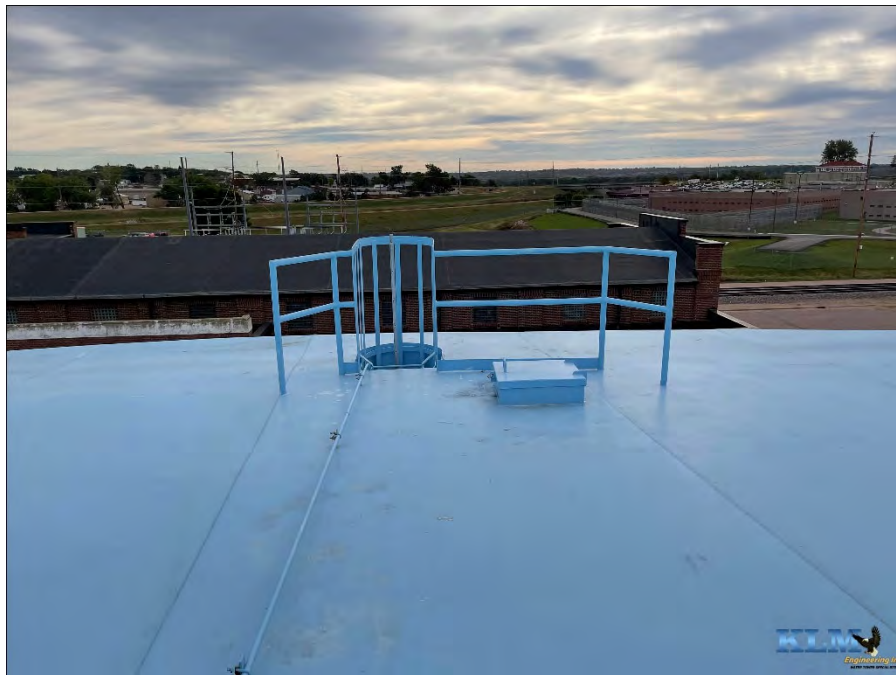
Photo No. 24 Roof ladder access and manway on roof
