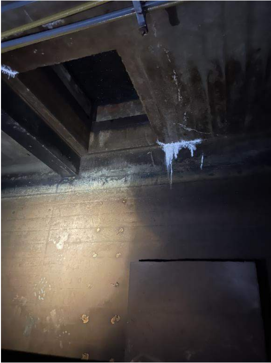
Figure 4 Mineral intrusion at crack in roof slab
