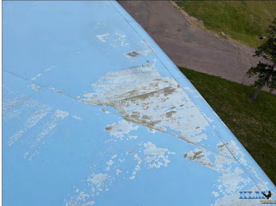
Photo No. 23 Coating conditions on roof
