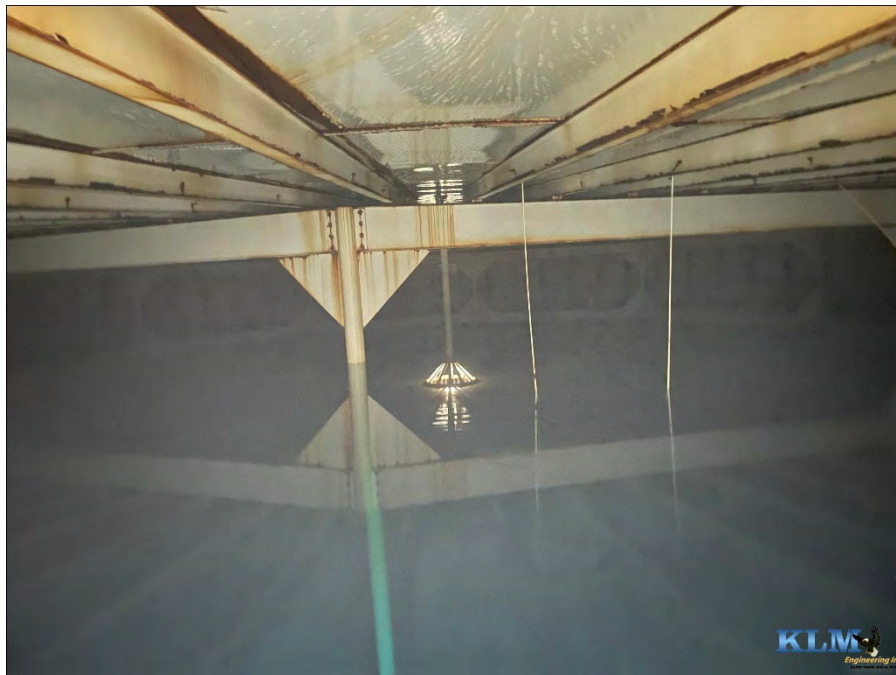
Photo No. 2 Interior conditions
