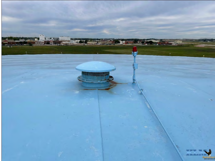
Photo No. 15 Overall roof conditions
