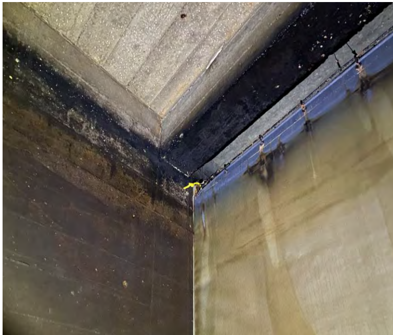
Figure 31 Baffle curtain (top connection)
