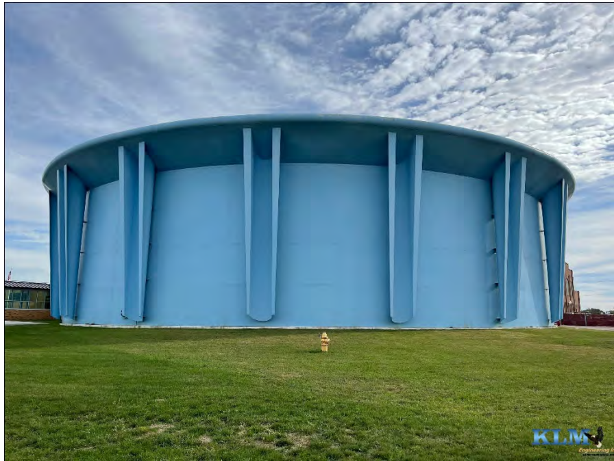
Photo No. 1 Overall view of reservoir
