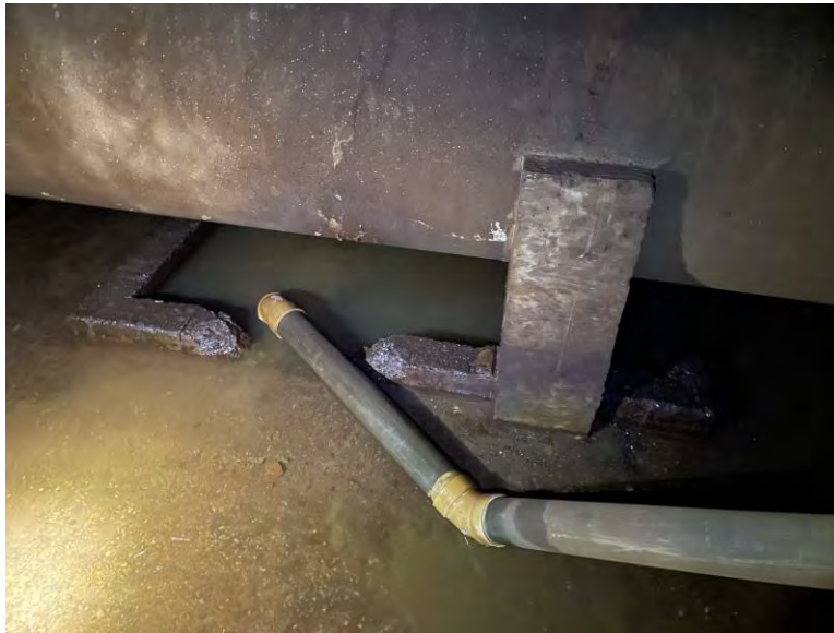
Figure 22 Drain pipe (sump location)
