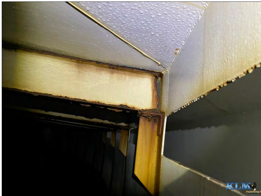
Photo No. 10 Condition of rafter connections
