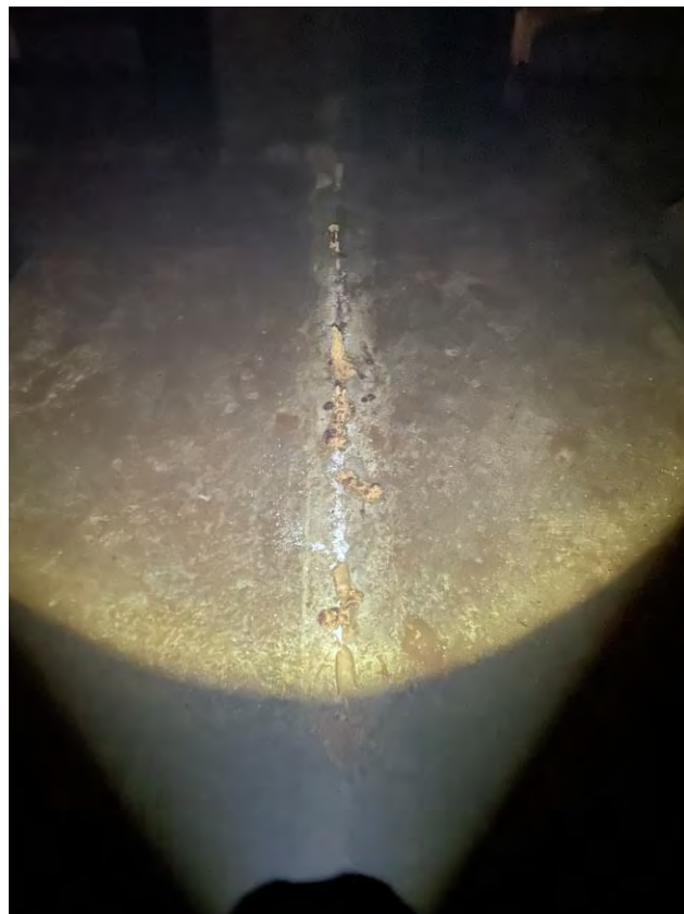
Figure 11 Joint sealant in mat slab
