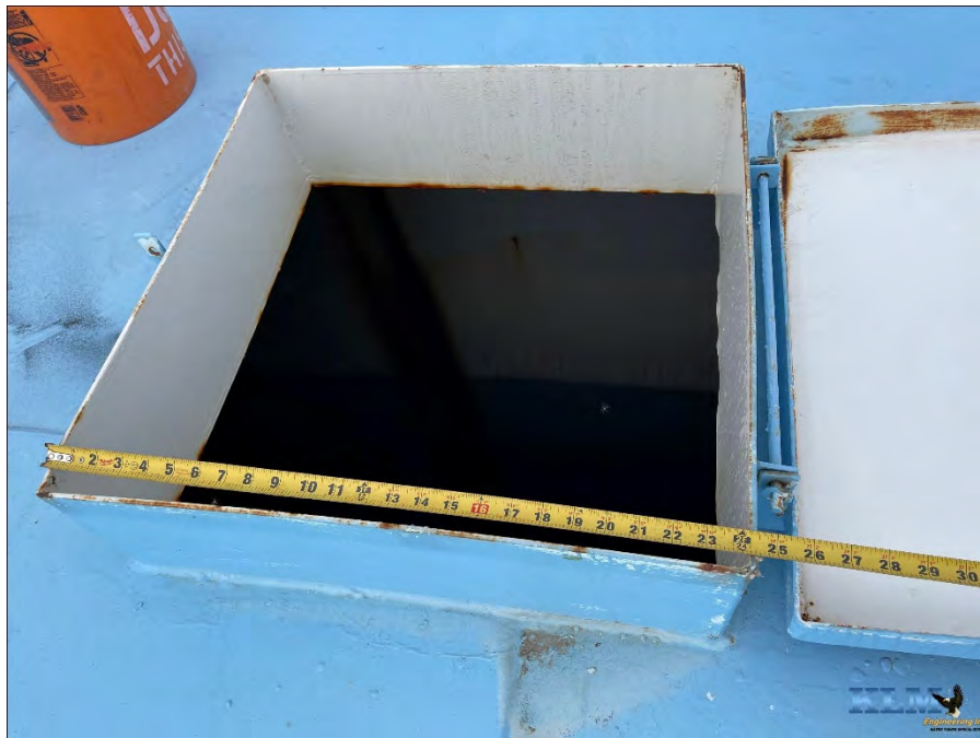
Photo No. 18 Manway condition
