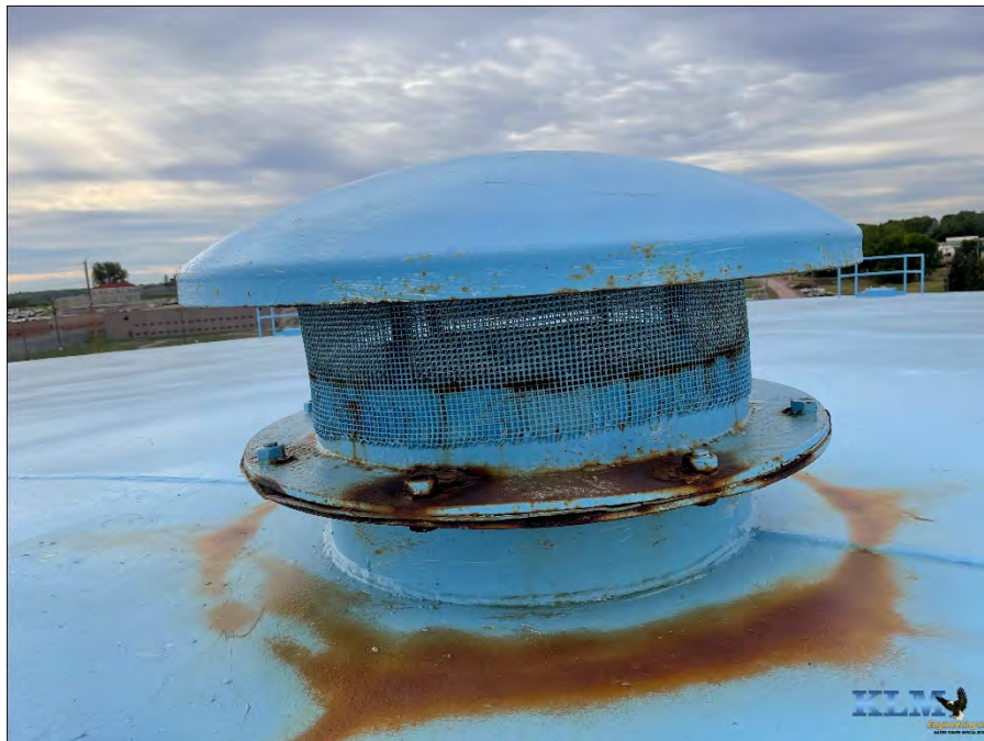
Photo No. 16 Roof and finial vent conditions
