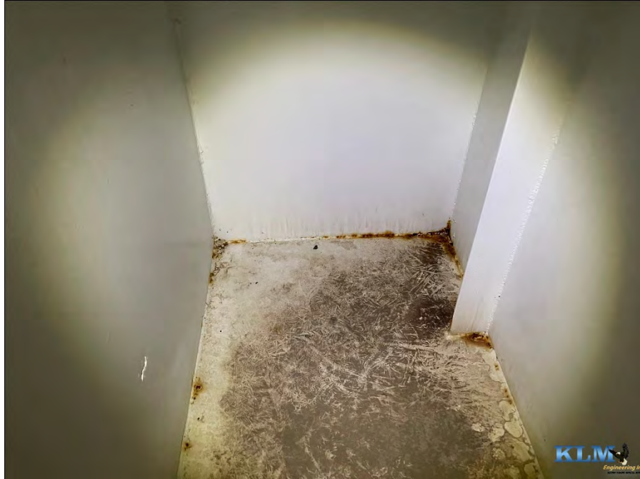
Photo No. 13 Overflow corridor condition
