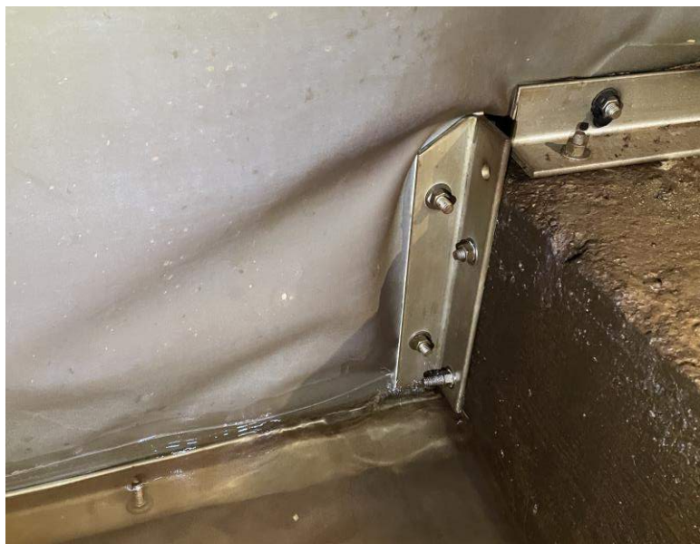
Figure 30 Baffle curtain (bottom connection)
