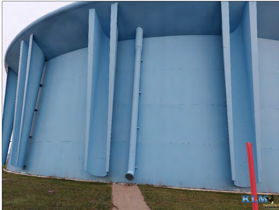
Photo No. 33 Overflow pipe on shell exterior
